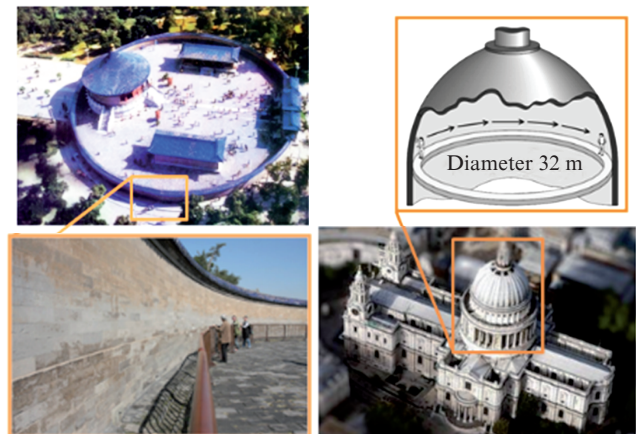
Figure 1. Echo Wall surrounding the Imperial Temple of Heaven (left) and the whispering gallery of St. Paul’s Cathedral in London (right).
